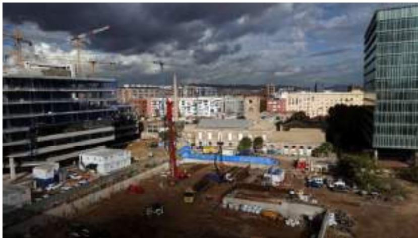
Figure 4 – Redevelopment work at Can Ricart
